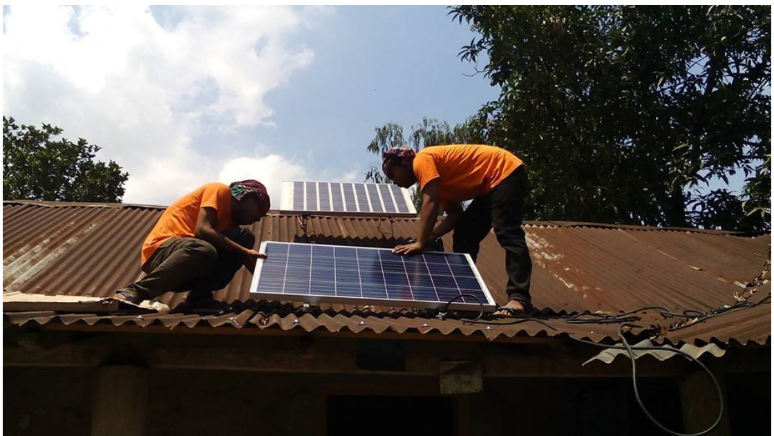
Figure 12: Installing solar panels in rural Bangladesh (Source: me-solshare.com)
