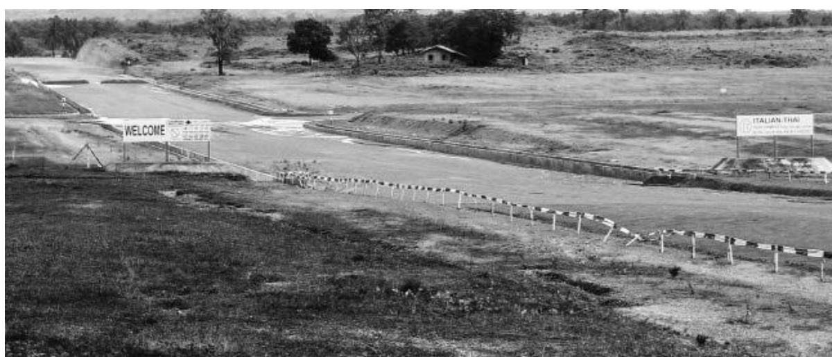
Figure 24: Road in DSEZ (Charlie Thame)
