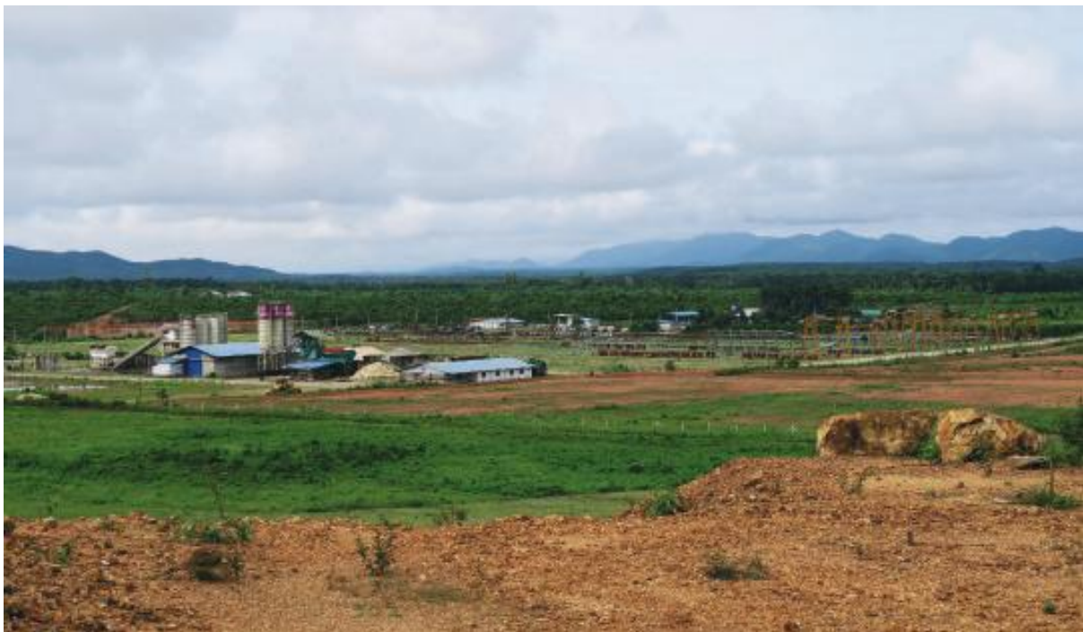
ITD worksite (July 2017) Photo by Ridan Sun
